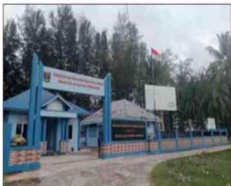
5. INSTALASI KKD BATANG GASAN
