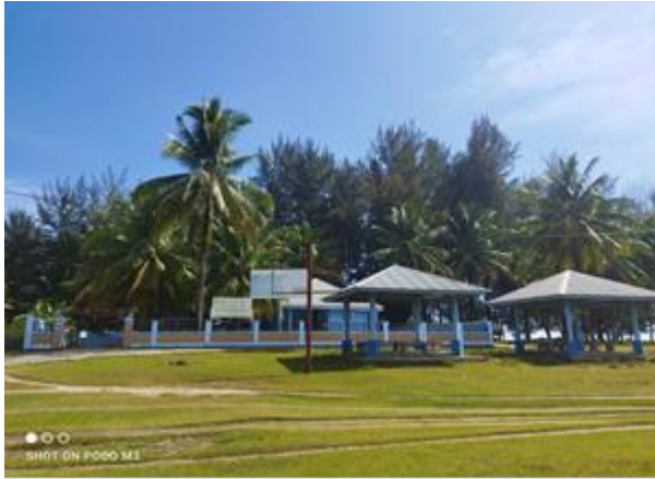
5. INSTALASI KKD BATANG GASAN
